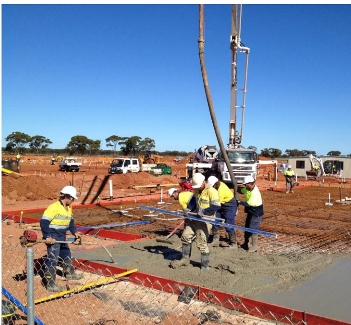
The first concrete ground slab is poured
