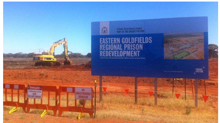
Work starts on new site next to existing prison.
